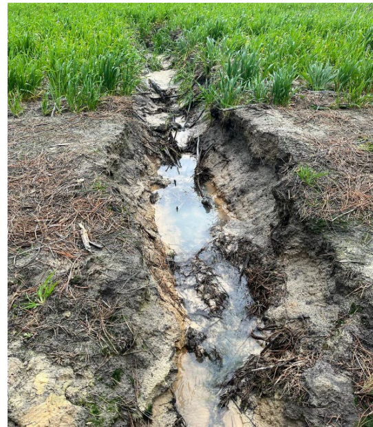
Figure 10. Localised erosion of the subsoil from the Dalyup subsurface drainage system. South Coast NRM 2024.
